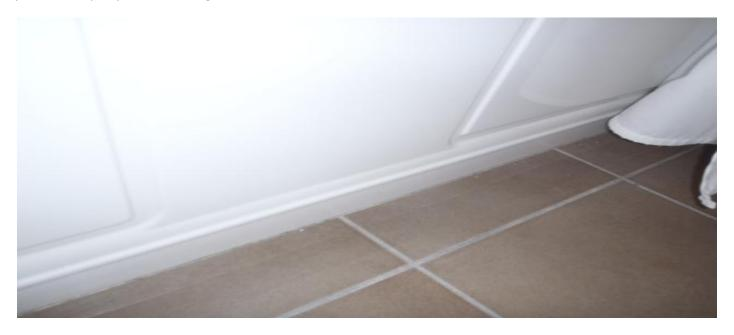
RE-CAULK THE TUB TO FLOOR JOINT IN THE BATHROOM. GROUT AND OR CAULK ALL VOIDS LOCATED IN THE BATHTUB AREAS TO PREVENT WATER MIGRATION INTO THE WALL SUBSTRATE.
