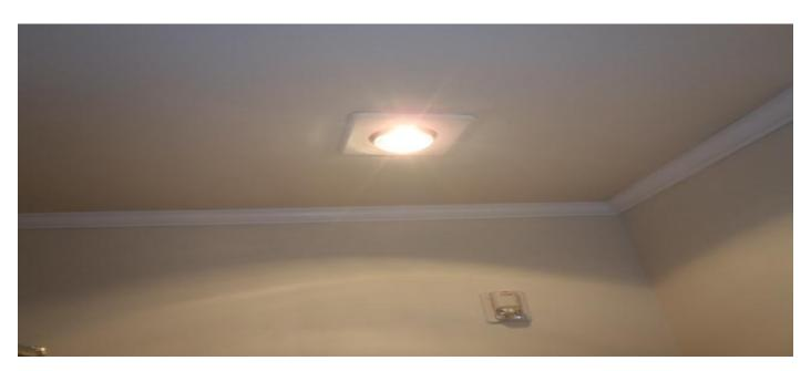
THE BATHROOM CEILING VENT FAN IS OUT OF BALANCE OR FAILING, COMPLETE ANY AND ALL REPAIRS FOUND TO BE REQUIRED TO ENSURE PROPER OPERATION.
