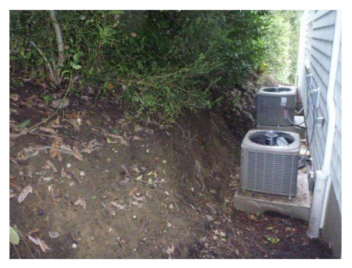
**Missing retaining wall:** A retaining wall system must be installed on any grade that is greater than 45 degrees of slope. A grade steeper than 45 degrees can be unstable and may slide. A retaining wall system must be installed to properly support the steep slope area.
