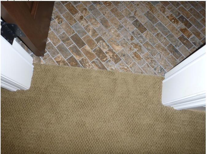
THE TRANSISTION AT CARPET TO STONE FLOORS IN THE BASEMENT SHOULD HAVE THE TACK BENT OVER. IF YOU ARE IN BARE FEET YOU WILL BE PUNCTURED BY THE TACKS.
