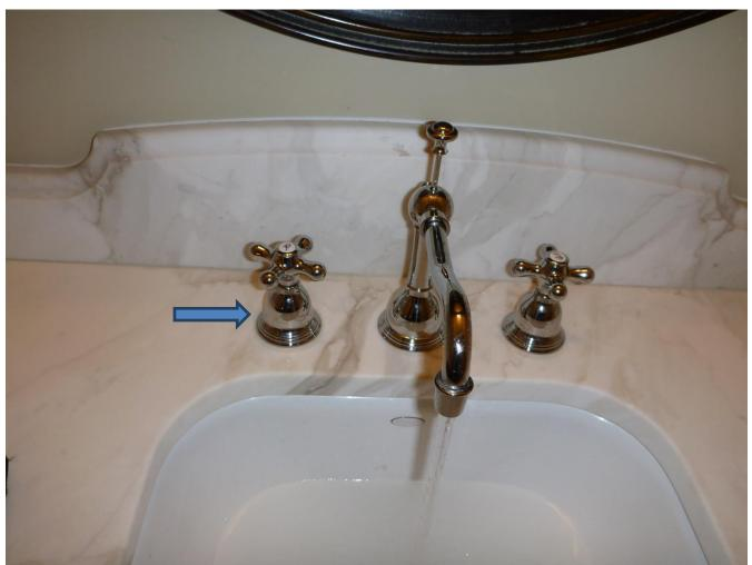
PROPERLY TIGHTEN THE HOT WATER CONTROL VALVE IN THE GUEST BATH, IT IS SPINING WHEN SHUTTING THE VALVE AND NEEDS TO BE TIGHTENED WITH A BASIN WRENCH FROM BELOW THE SINK.
