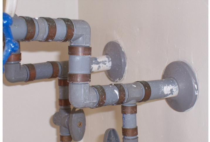
tures result, and the basic structural integrity of the system is reduced. Thus, the system becomes weak and may fail without warning causing damage to the building structure and personal property. It is believed that other factors may also contribute to the failure of polybutylene systems, such as improper installation, but it is virtually impossible to detect installation problems throughout an entire system.
