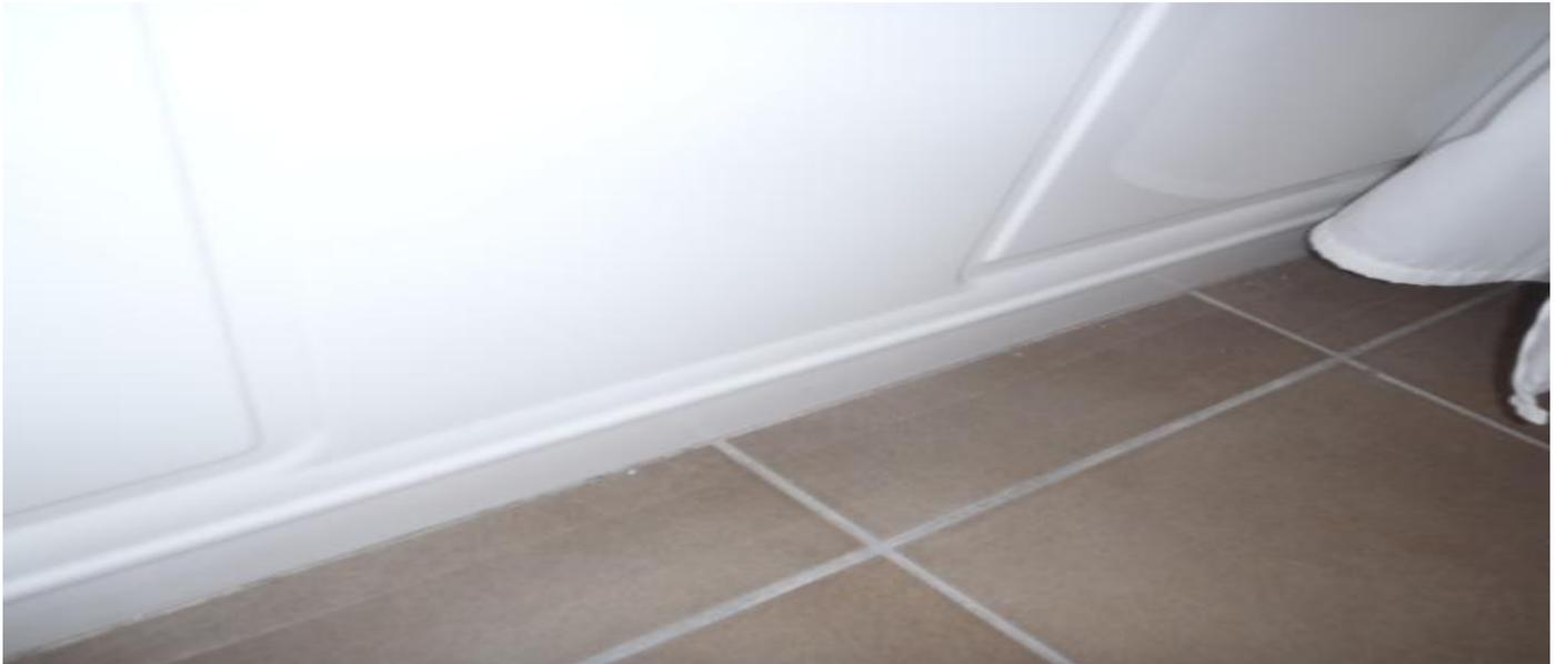
**RE-CAULK THE TUB TO FLOOR JOINT IN THE BATHROOM. GROUT AND OR CAULK ALL VOIDS LOCATED IN THE BATHTUB AREAS TO PREVENT WATER MIGRATION INTO THE WALL SUBSTRATE.**
