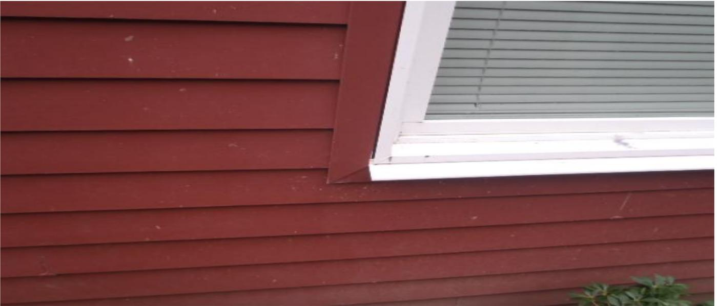
**RE-CAULK ALL FAILING CAULKING AS LOCATED AT THE SIDING BUTT ENDS, FACE NAILING, WINDOW AND TRIM SYSTEMS AND AS FOUND TO BE REQUIRED TO PREVENT WATER MIGRATION INTO THE SIDING MATERIAL AT ALL SIDES OF THE STRUCTURE.**
